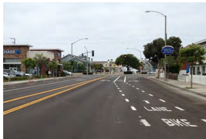
Roadway reconfiguration to provide bicycle lanes. (Source: City of Newport Beach)
